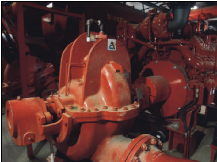
Each of the skid-mounted pumps from A-C Custom Pump are designed to deliver fire-quenching water at 5,000 gallons per minute.
